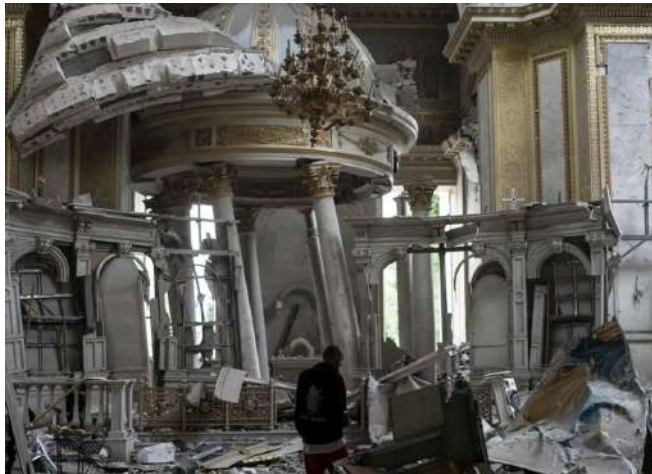
The drone attack wreaked extensive damage to the cathedral
