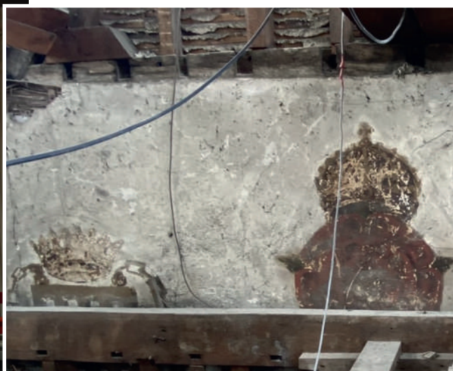
A series of rare medieval wall paintings have been uncovered by builders working in a roof space at Christ's College, Cambridge University. They are believed to date from the 16th century
